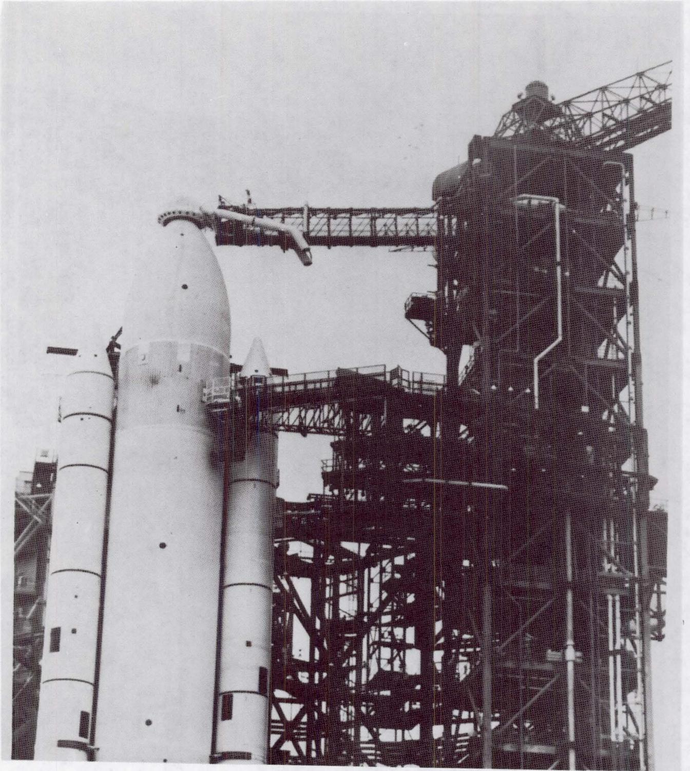
Figure 6. ET GOX Vent System Installed at Pad 39A for STS-2 Launch
