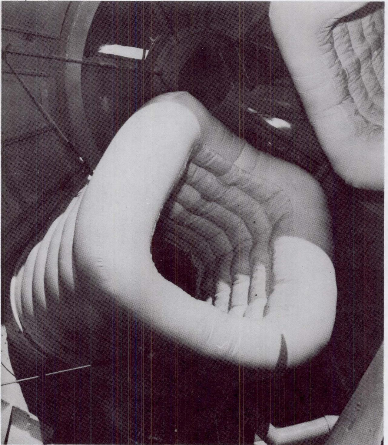
Figure 4. ET GOX Vent Inflatable Seals
